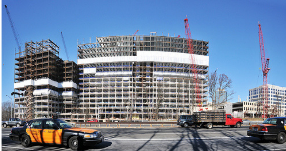
Precast exterior wall panels are quickly rising to the top of 17-story and 15-story office towers as construction continues on the $1.8 billion Department of Defense Office Complex (BRAC 133) at Mark Center in Alexandria, Va. The Corps' New York District is managing design and construction of the project, which will relocate around 6,400 Defense Department employees from leased office space in the region to a single campus in Alexandria. Photo Credit: Marc Barnes, Belvoir Integration Office Public Affairs.
